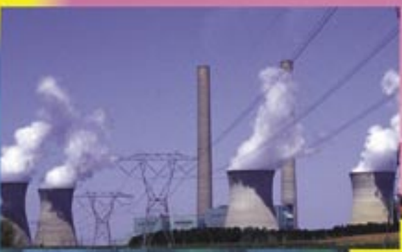
Georgia Power's Plant Bowen, located near Cartersville, Ga., is one of the country's top electricity-producing power plants. The four coal-fired units supply power to Georgia over 500kv high-voltage transmission lines like shown here.
