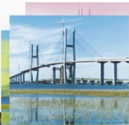
The Sidney Lanier Bridge near Brunswick, Ga., one of America's ten largest bridges, has 485-ft towers and 7,781-ft. total length. This cable-stayed design bridge is an architectural masterpiece of Structural Engineering. It was jointly funded by the State of Georgia and the U.S. Coast Guard.
