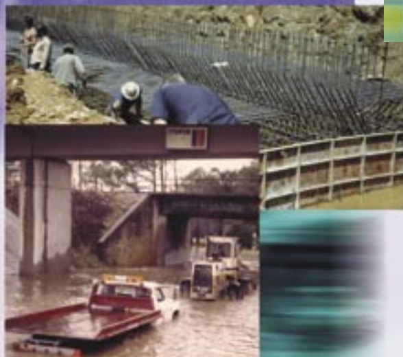
Civil Engineers design structures to prevent problems such as this, seen near Atlanta, Ga. Courtesy of Rufus O. Terrill, PE, Terrill Technologies, Inc., Atlanta, Ga
